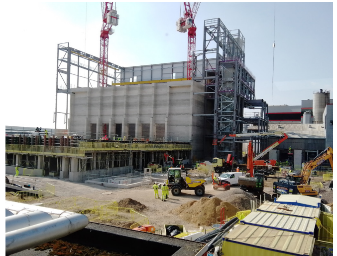
The Slough Multifuel project currently under construction
