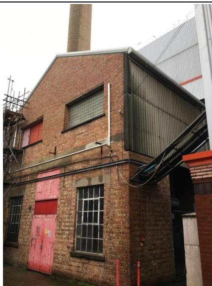
Photograph 4: B26 with corrugated asbestos sheeting providing crevices (potentially suitable roost features).
