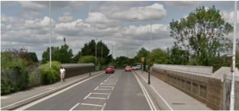
Farnham Road Overbridge Approx. 35m in length, Bollards 7m <> and speed camera.
