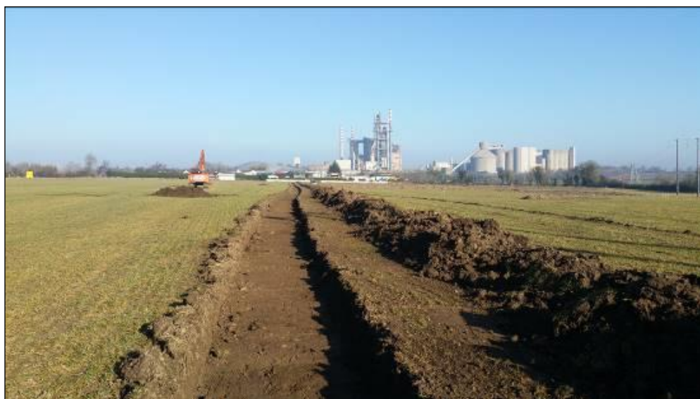
Plate 4: Test Trench 15 – looking N towards Irish Cement Works facility
