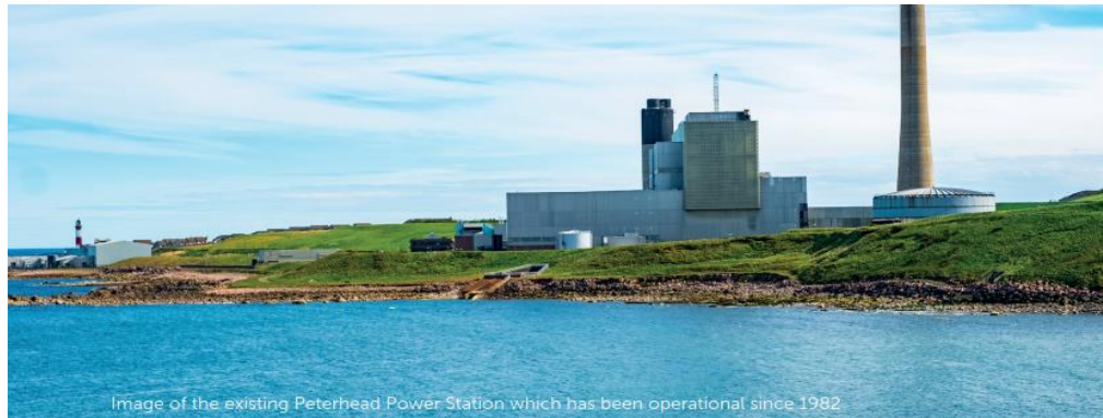
Image of the existing Peterhead Power Station which has been operational since 1982
