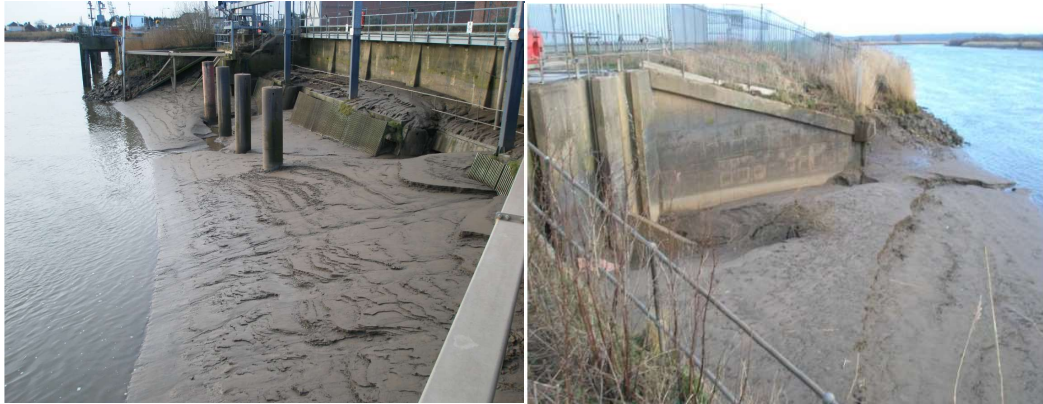
Diagram 2: Keadby 1 Power Station intake (left) and outfall (right) taken during outage
