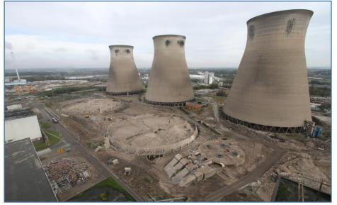
Keltbray successfully carried out the explosives demolition of 4No Cooling Towers on 13<sup>th</sup> October. The works were a year in the planning, 4 months preparation and took approx 12 seconds to fall.
