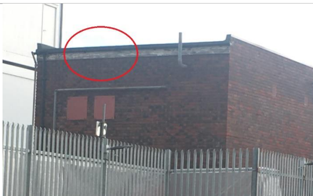
Photo 4. Gap in under bargeboard (F005) in B3
