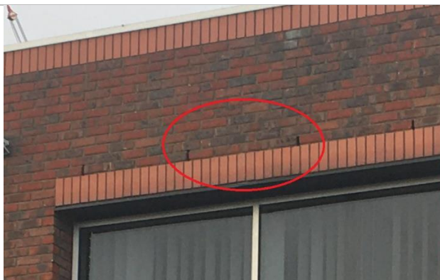
Photo 6. Shallow gaps in brickwork (F007) in B5
