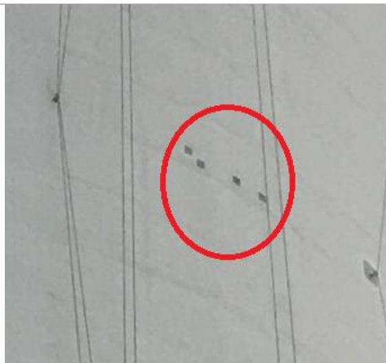
Photo 1. Ventilation gaps in concrete (F001) in B1
