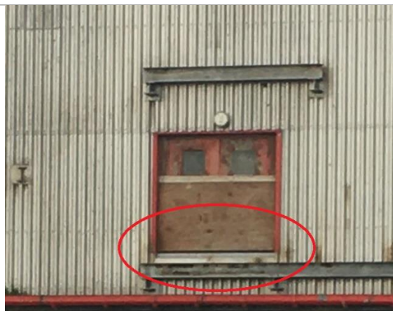
Photo 5. Gap behind plywood (F006) in B4
