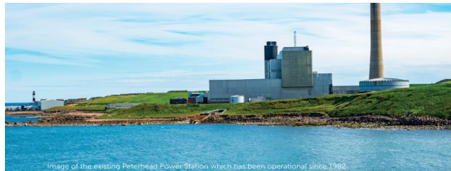
Image of the existing Peterhead Power Station which has been operational since 1982.
