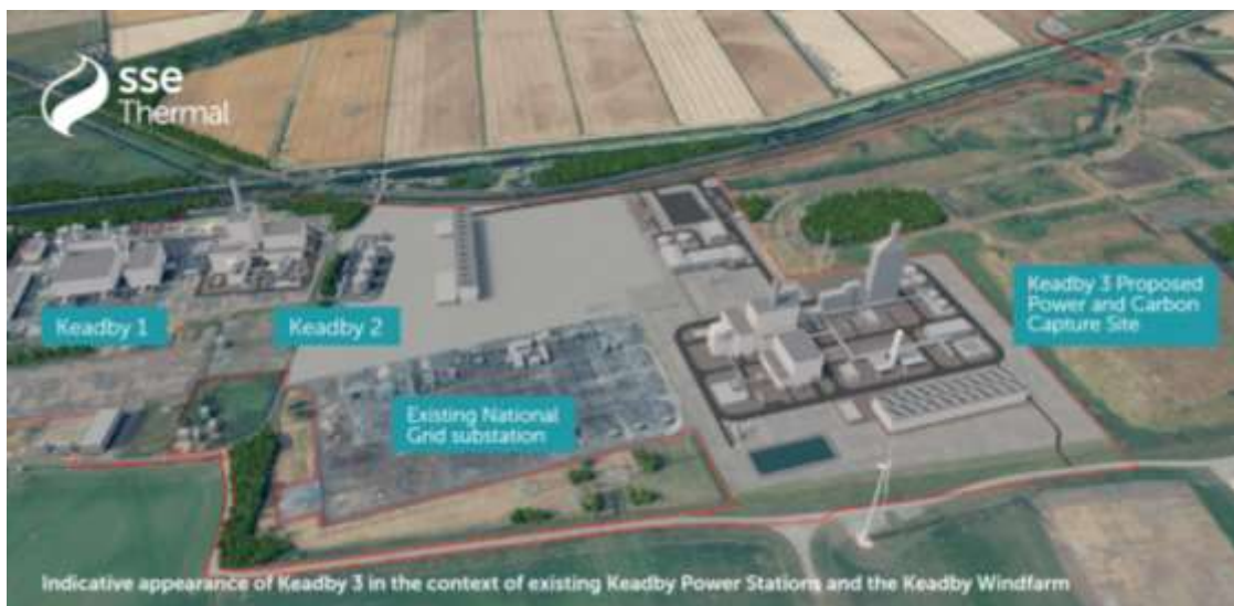
Figure 3.2: Indicative 3D rendering of the Proposed Development within the Keadby Power Station site
