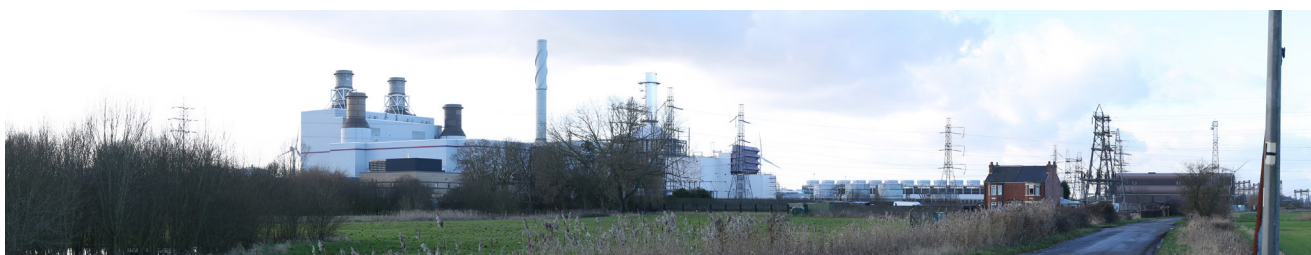
Existing view along Chapel Lane (winter)
