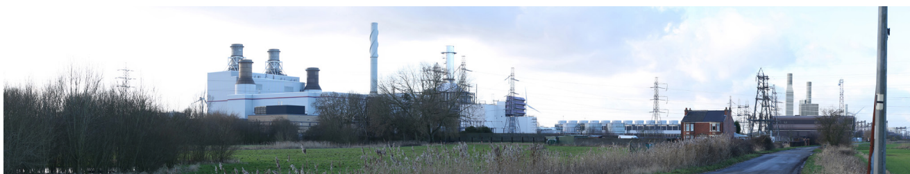
View along Chapel Lane (single absorber with taller carbon dioxide stripper)
