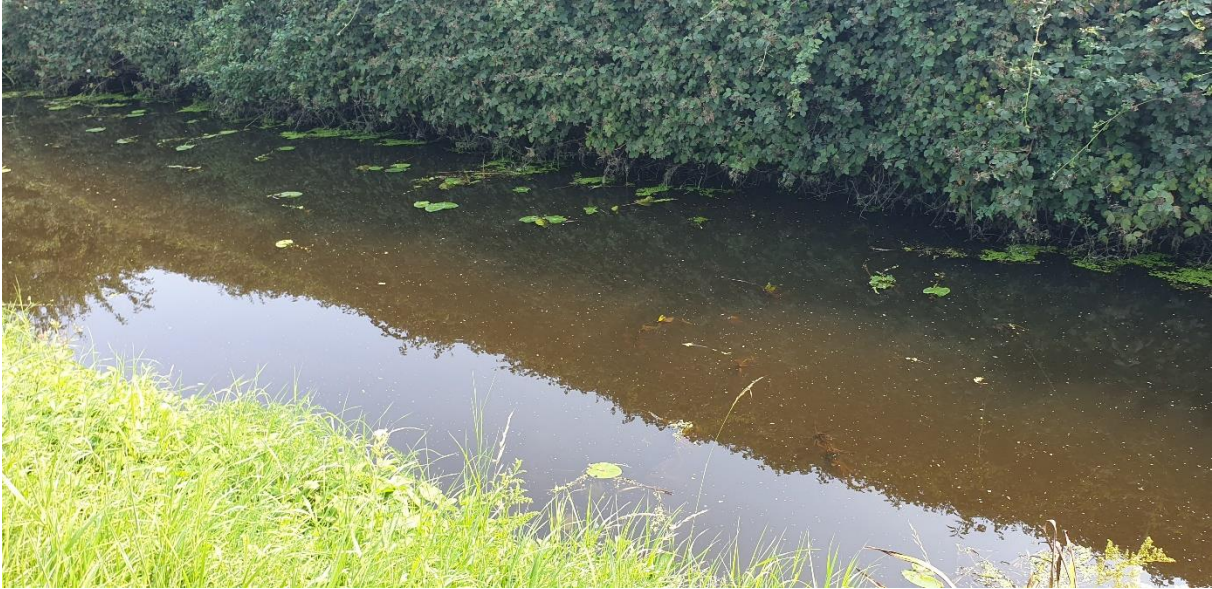
Photograph 7 – North Soak Drain
