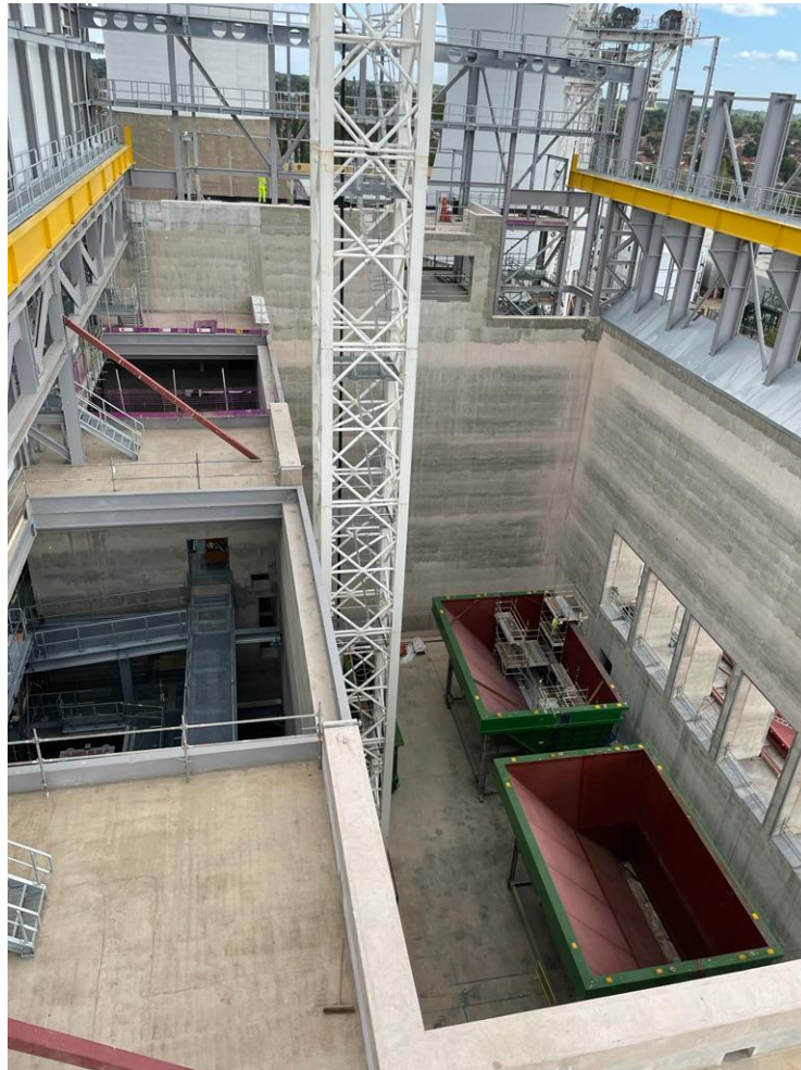
Plate 4.4 – Feed Hopper Openings Consented Development Construction Works (August 2022)
